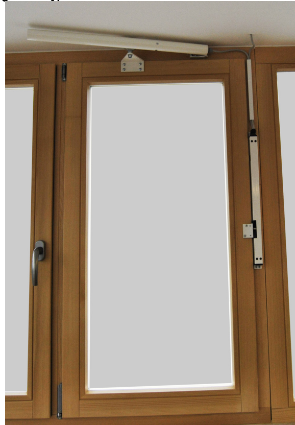
Figure 6: Typical Installation with slit actuator
